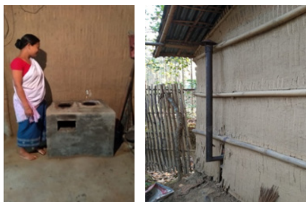
Homemaker with cook stove and chimney
